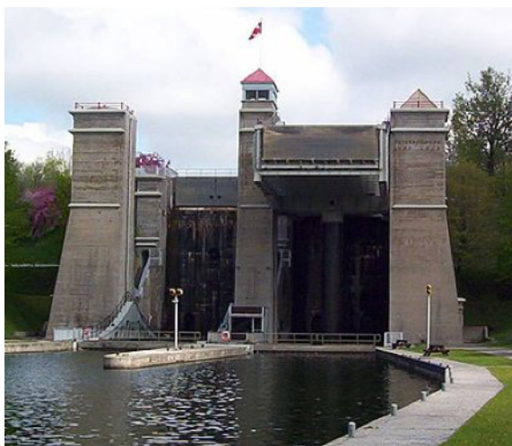
Photo 2: Hydraulic lift lock on the Trent-Severn.
