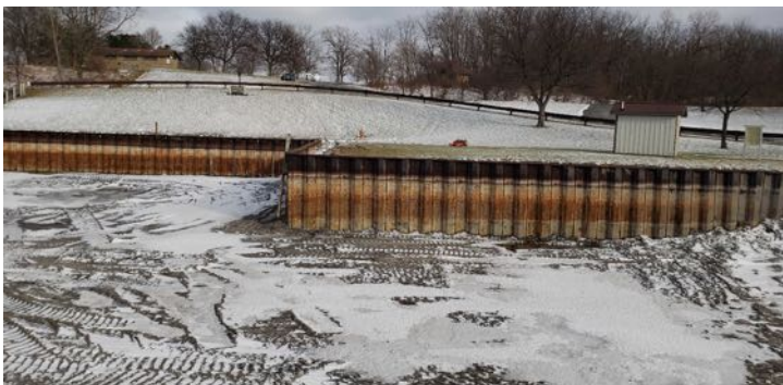
Photo 4: After dewatering and “dredging” the marina.
