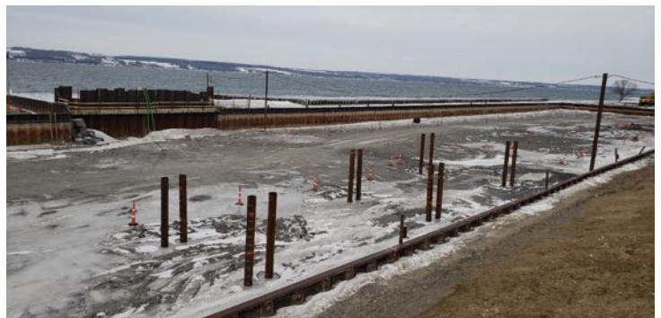
Photo 5: The temporary “dam” in place that allowed dewatering, “dredging” and reconstruction work. New dock structural supports being installed.
